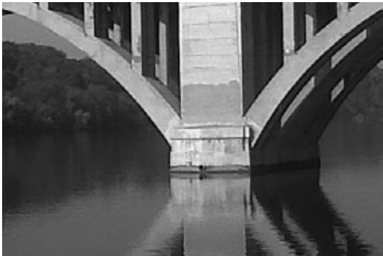
Key Bridge again a beautiful site (photo by Walter Groszyk)
