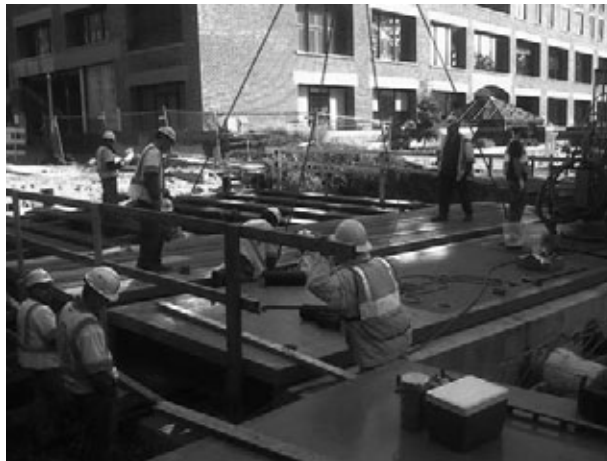
Installing the fiberglass bridge deck on the 29th Street bridge
