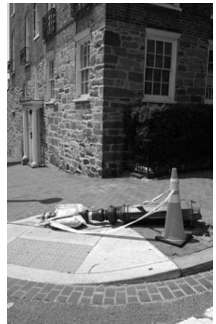
The historic call box toppled by a GUTS bus at 34th and Prospect was rescued by the BID, DPW and John Dreyfus. GU is working on the repair and installation.
