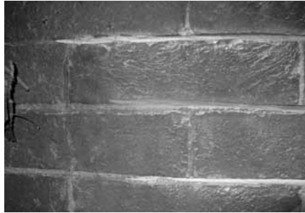
Power saw damage on bricks.
