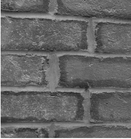
An example of poor repointing.
